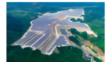
Mega solar power plant in Kurokawa District, Miyagi Prefecture
