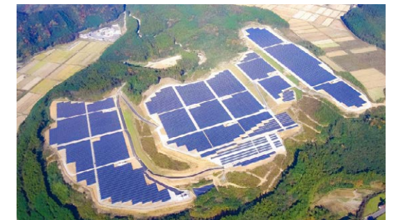
Jointly operated mega solar power plant in Hagi City, Yamaguchi Prefecture
